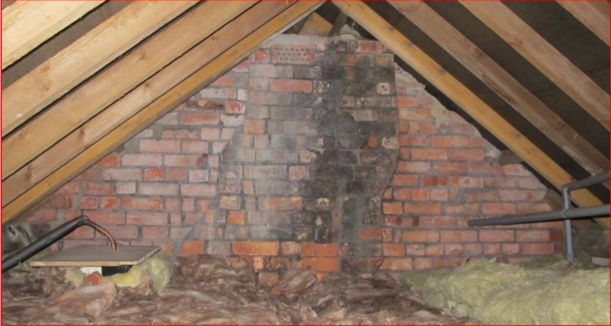
Solid Party Wall – Solid brick showing clear stretchers and headers.
