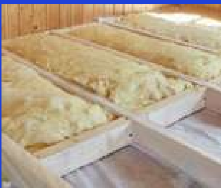
Mineral Wool - 0.040 \text{ W/m}\cdot\text{k}
