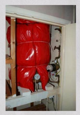
3) Jacket insulated: Jackets are very simple to identify and are usually coloured red. The process for assessing a jacket's insulation is the same as foam insulated cylinders.
